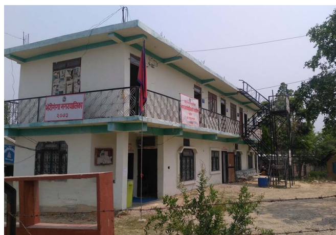
Bheriganga Municipality office building
