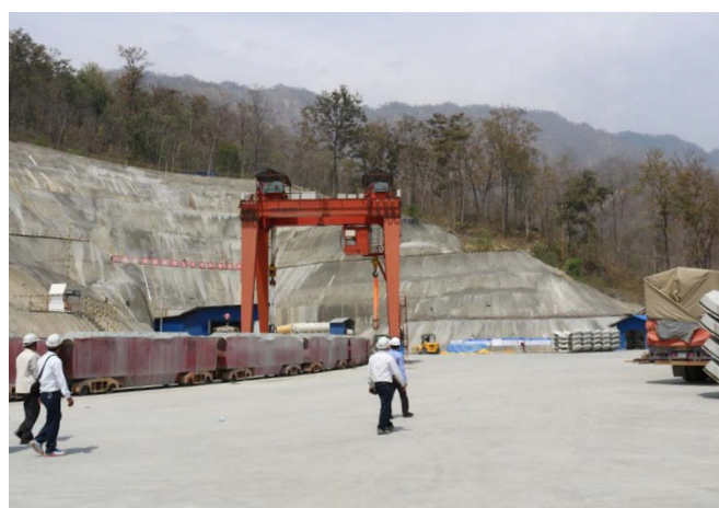
Bheri-Babai Tunnel Construction
